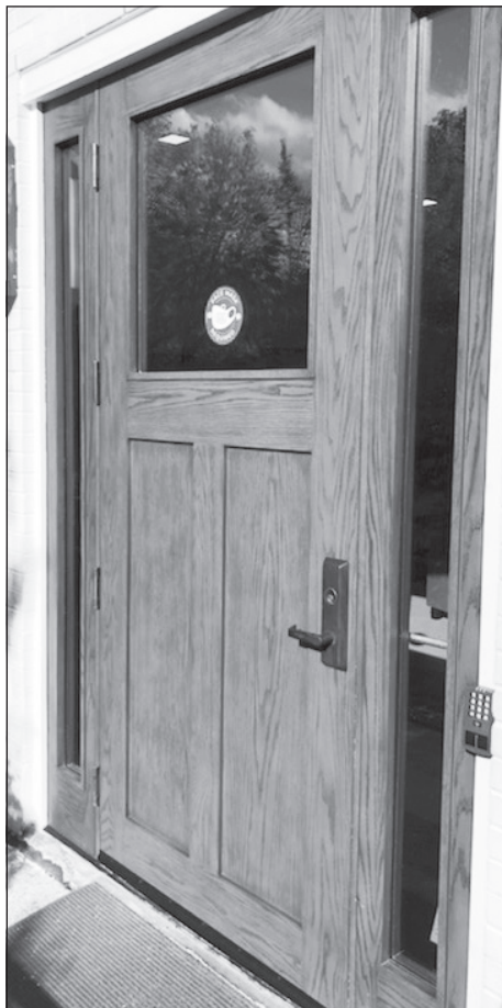
Installation of New Kitchen Door
